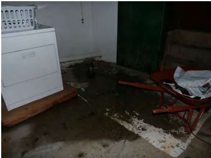
Example of water infiltration noted at several unit basements
