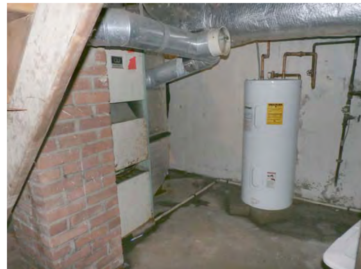
Typical heating furnace and domestic hot water heater
